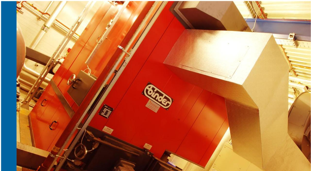
**Narec installed a biomass boiler at its former high voltage testing laboratory in Hebburn to help reduce annual energy costs and carbon emissions.**
